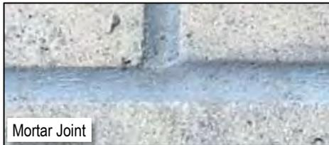
Tooled mortar joints are best suited for masonry-bound trim items such as belt courses, lintels, window surrounds, date stones, inscription blocks, quoins, keystones and similar applications. Rake and point the mortar joints rather than full-bed setting and finishing in one operation. See Technical Bulletin #44 on Pointing.
