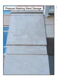
Direct high pressure power washing and sandblasting are not recommended procedures for cleaning cast stone. Furthermore, metal fiber brushes, rubbing stones and any tool or device that can scar the cast stone not to be used for cleaning cast stone.
